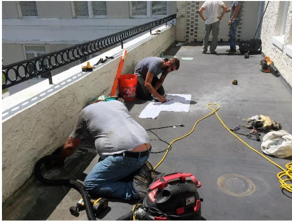
Workers level low spots on the surface
