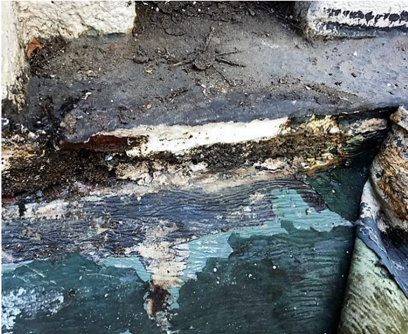
Water was under the lowest roof layer that was meant to be water-proof. This degrades the concrete, and causes leaks
