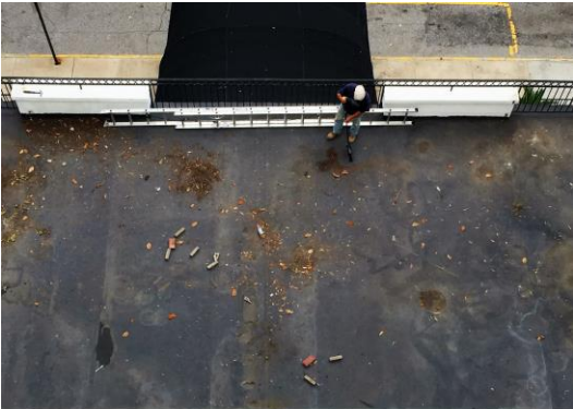
Railings were removed from roof. Note worn surface
