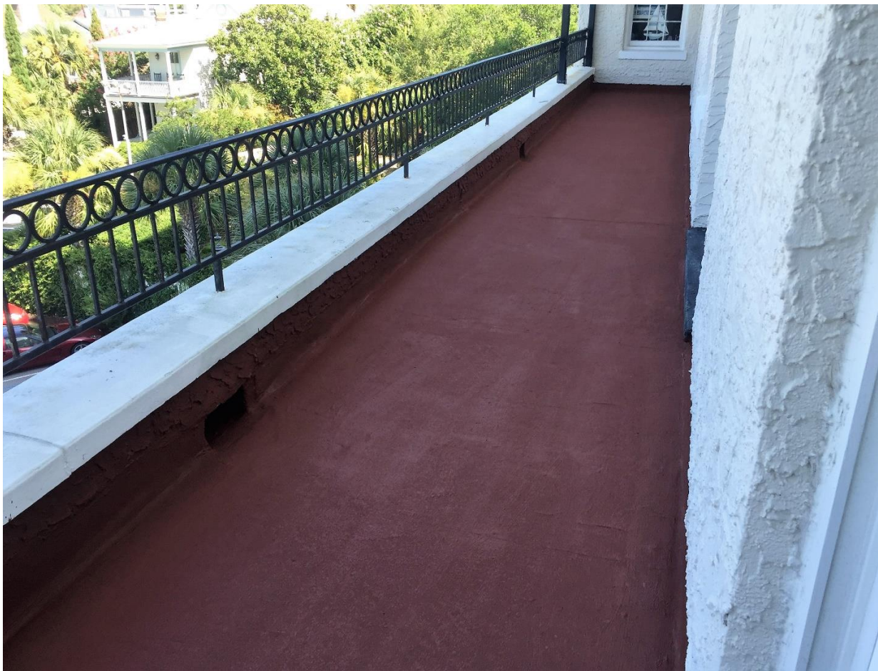
The finished surface—six layers---terra cotta color
