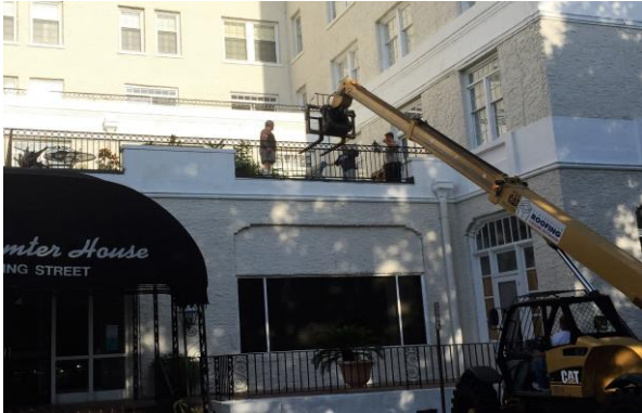
Removing everything from the roof
