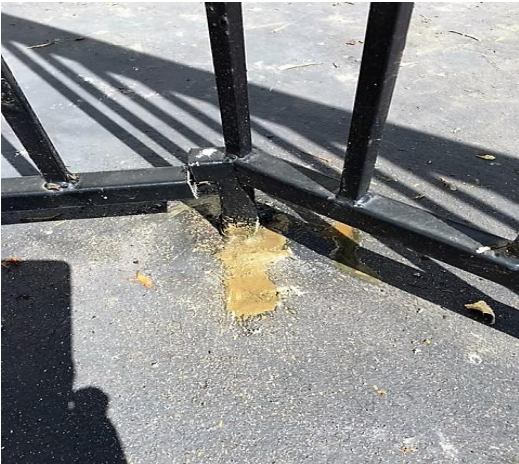
Water was in the railings, causing rust and leaks
