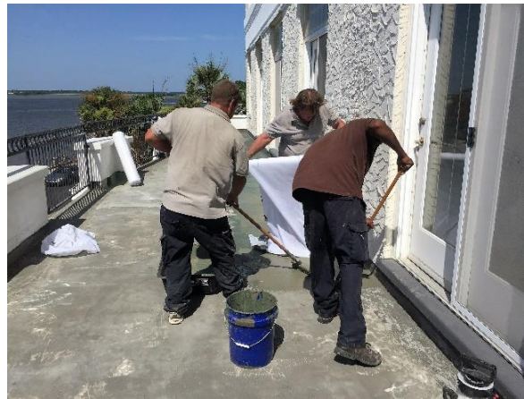
Workers install the first two layers of new roof coating
